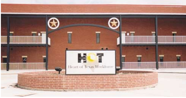
Heart of Texas Workforce facility, under construction - Waco, Texas.
